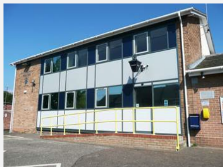
THETFORD POLICE STATION RETAINED
