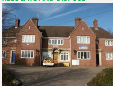
ACLE POLICE STATION RELOCATE AND DISPOSE
