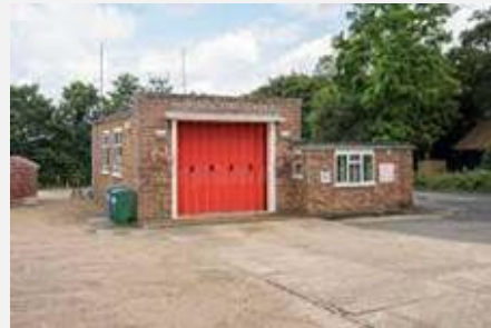
LODDON FIRE STATION REVIEW FOR POLICE USE
